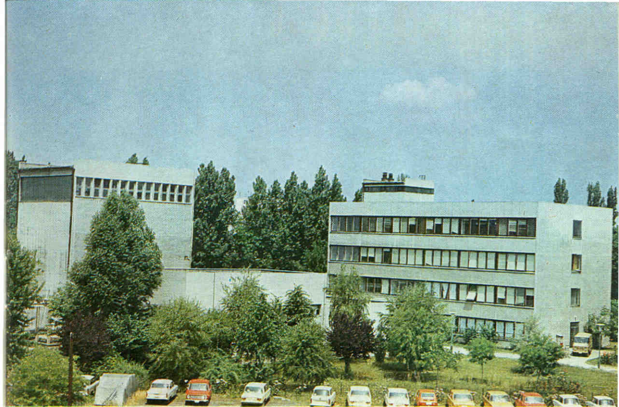
Buildings erected in 1971
